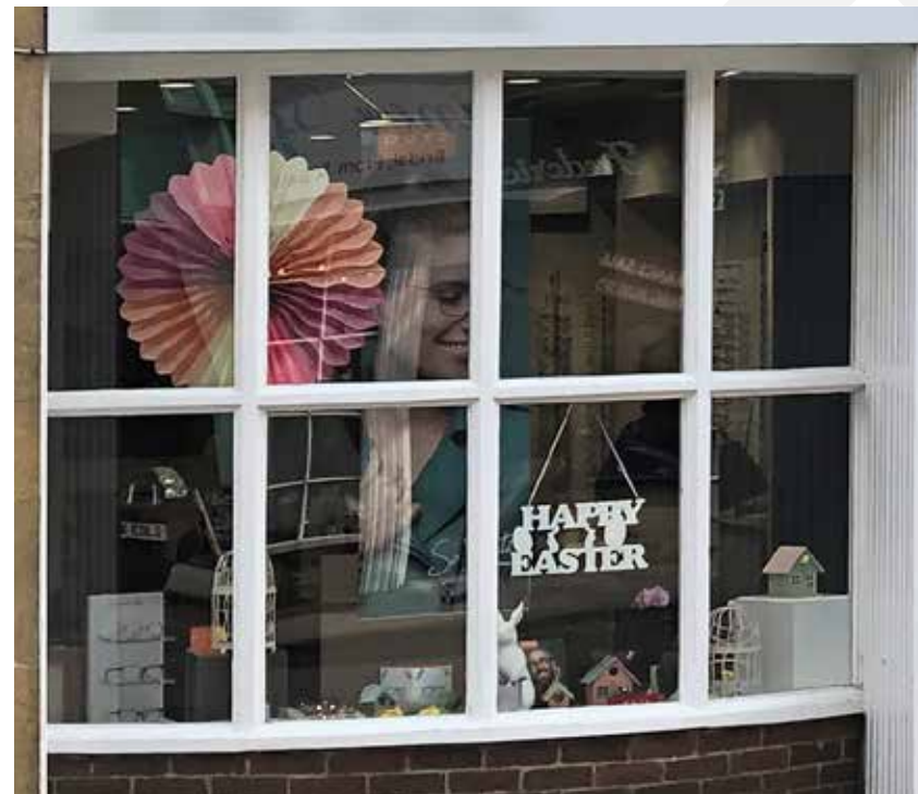
Figure 20. Timber mullions and transoms subdividing shopfront display
