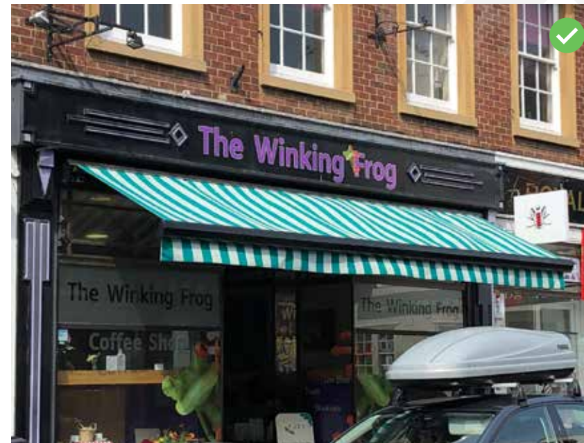
Figure 44. Well integrated retractable blind
