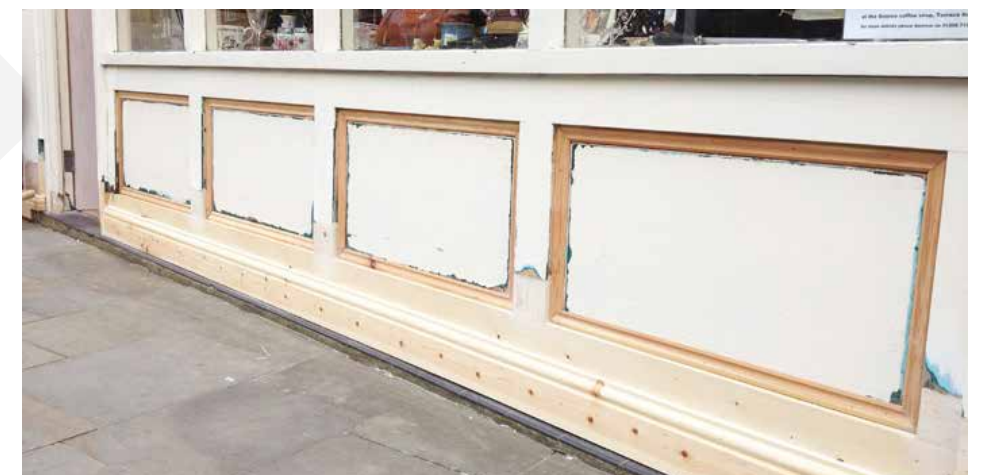
Figure 56. Timber stallriser repair
