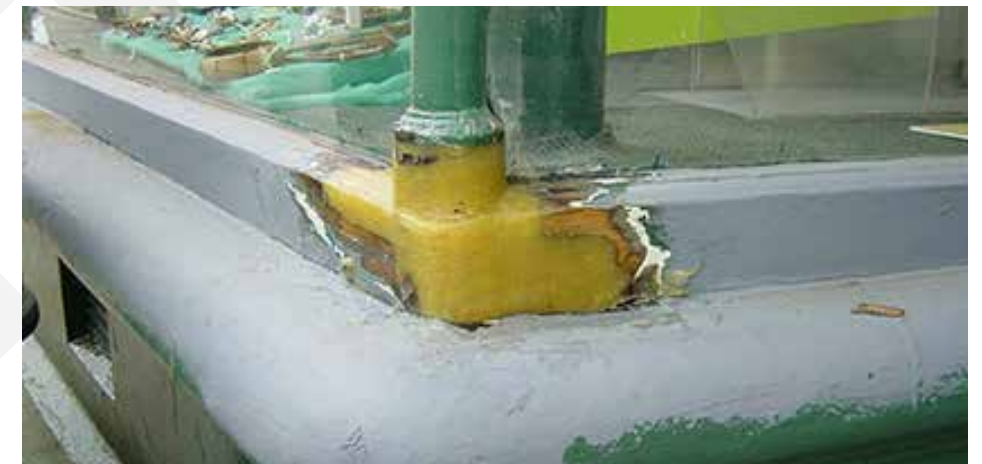
Figure 55. Resin repair to timber shopfront detail
