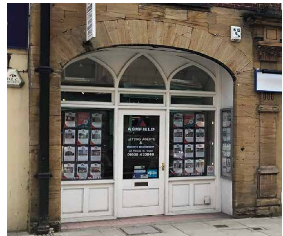
Figure 25. Recessed doorway, shopfront style matches building setting, panelled stallriser
